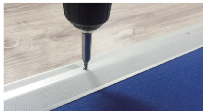
4. Screw fixing 紧固螺丝
