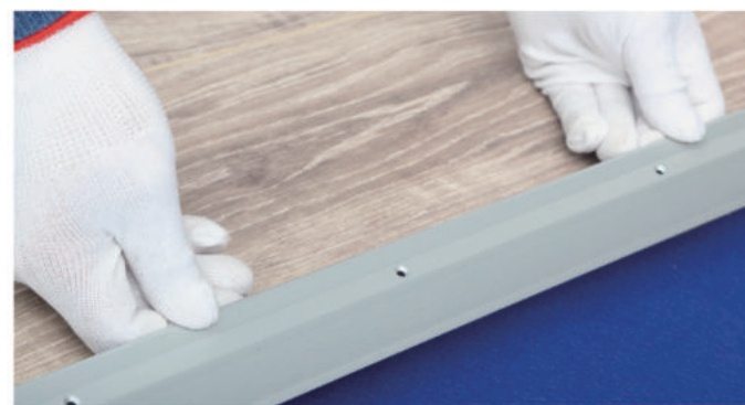
3. Install base profile &amp; put cover profile 安装底座并放上盖板
