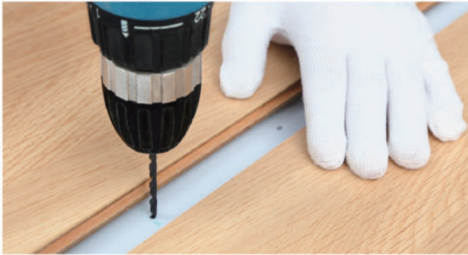
1. Hole positioning & drilling 孔定位并钻孔
